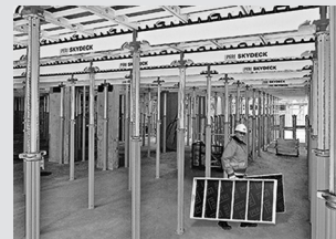
Slab formwork
