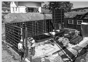
Wall formwork
