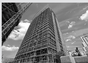
Working scaffolds for facades
