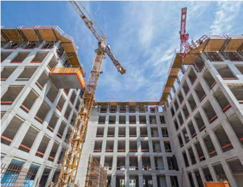
The Folding Platform System FB 180 served as a working and formwork scaffold for the office and hotel building. An RCS MP Landing Platform could be positioned freely in order to relocate and temporarily store formwork material.
