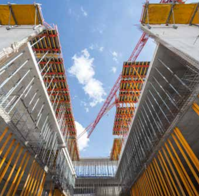
The Folding Platform FB 180 together with the MAXIMO Wall Formwork ensured that the strict tempo specifications could be met.
