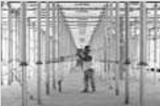
Slab Formwork
