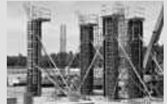
Column Formwork
