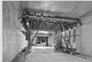
Tunnel Formwork
