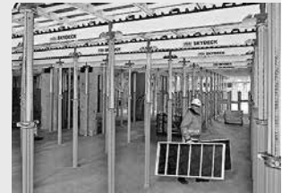
Slab Formwork
