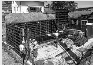
Wall Formwork
