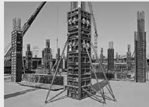
Column Formwork
