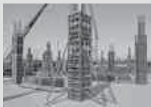
Column Formwork
