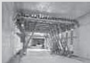
Tunnel Formwork
