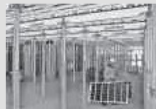
Slab Formwork
