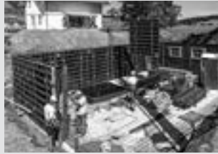
Wall formwork
