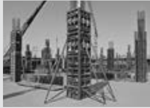
Column formwork
