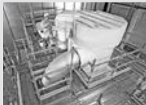
Working scaffolds industry
