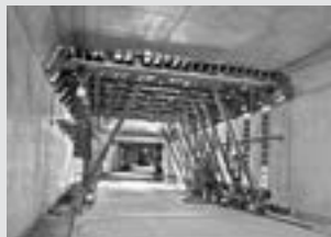
Tunnel formwork
