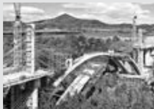
Bridge formwork
