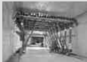
Tunnel Formwork
