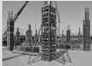
Column Formwork
