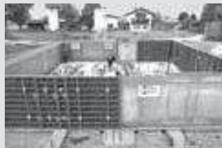
Wall Formwork
