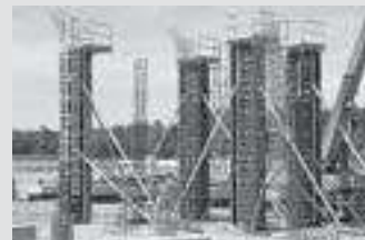
Column Formwork
