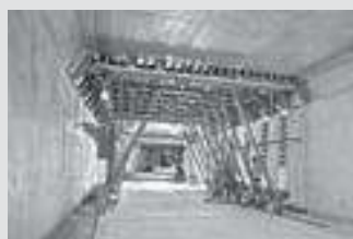
Tunnel Formwork
