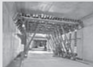
Tunnel Formwork
