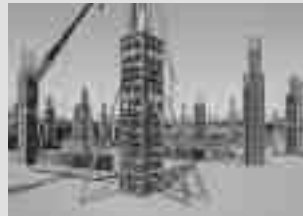
Column Formwork
