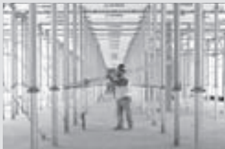
Slab Formwork
