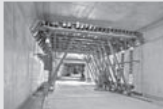
Tunnel Formwork
