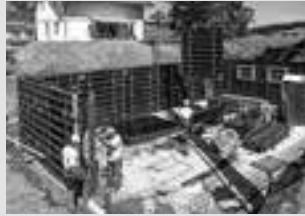
Wall Formwork
