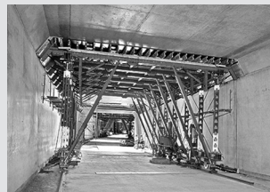
Tunnel formwork
