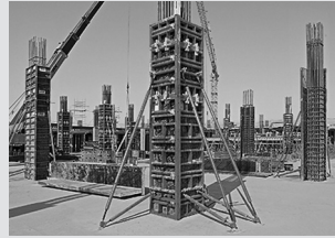
Column formwork
