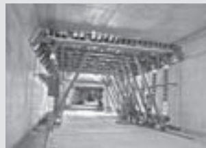
Tunnel Formwork
