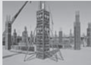
Column Formwork
