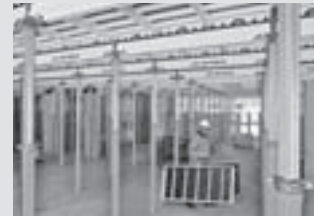
Slab Formwork
