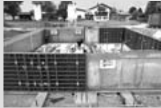
Wall Formwork
